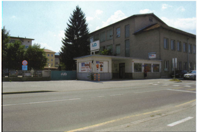
Figure 6. TVT Boris Kidrič, once producer of rail vehicles and heating devices in Maribor.
